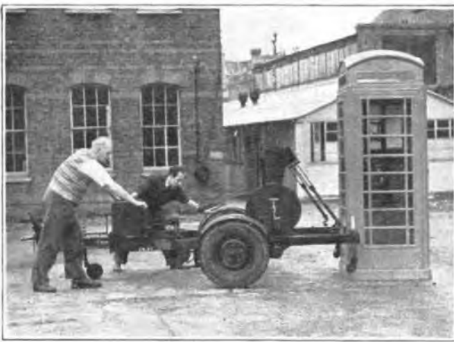
FIG. 1.—PLACING TRAILER AROUND KIOSK.
