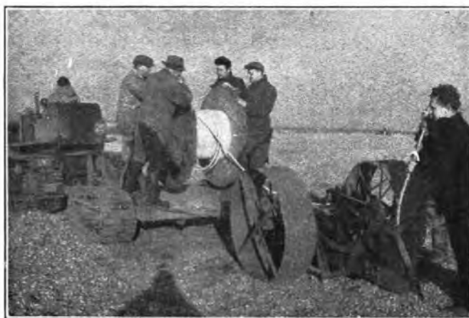
MOLEDRAINING CABLE IN SHINGLE.
