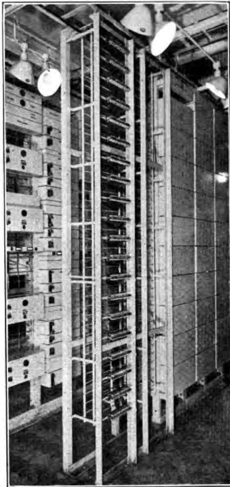
FIG. 13.—G.D.F. AND THROUGH-GROUP FILTER BAYS.
