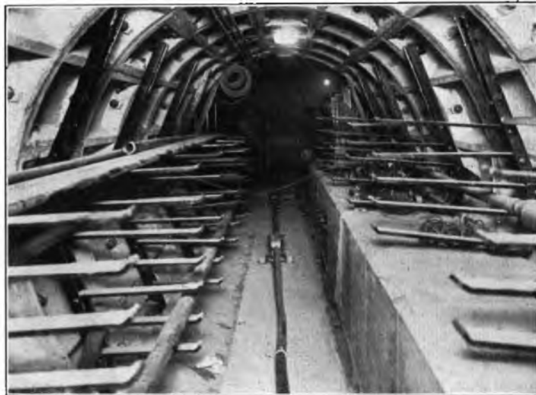
FIG. 6. CABLING OPERATIONS IN HOLBORN TUNNEL.
