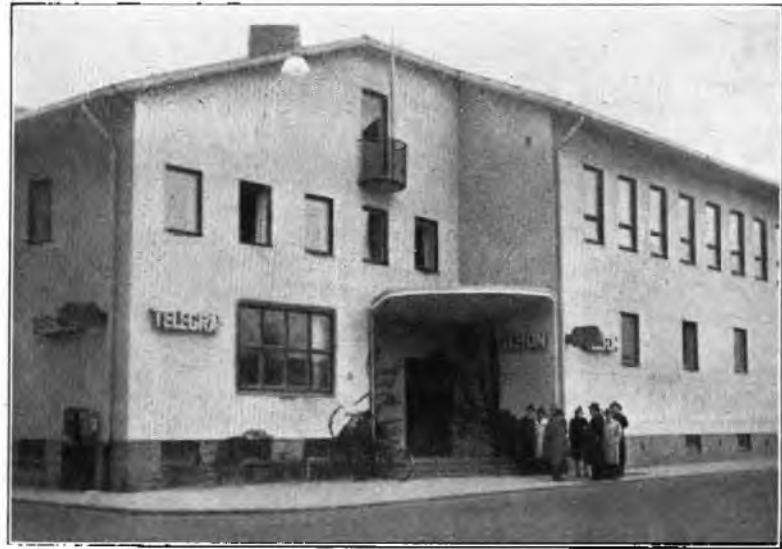
FIG. 2.—TELEGRAPH AND TELEPHONE BUILDING IN KRISTIANSTAD.
