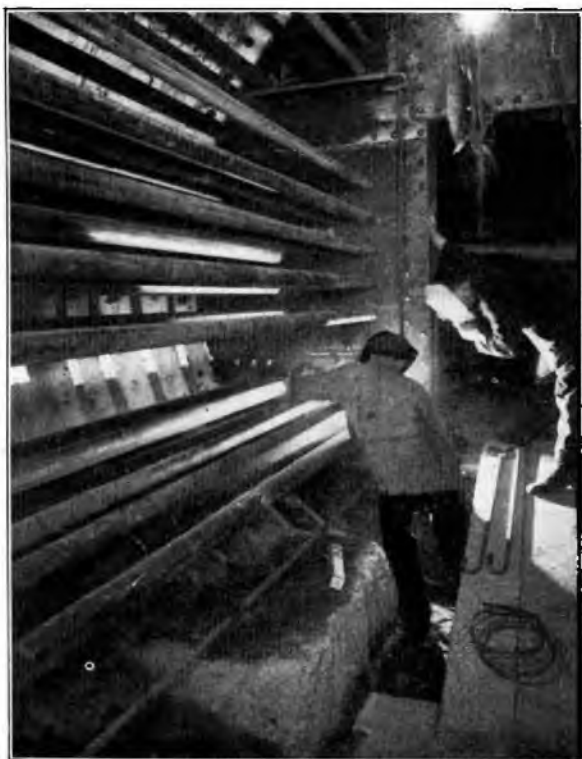
FIG. 1.—CABLE PIPES BEING WELDED TO MAIN PLATE OF BULKHEAD.
