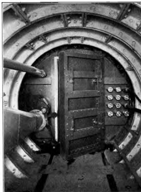
FIG. 2.—COMPLETED BULKHEAD IN 8 FT. DIA. LATERAL (VIEW FROM FOOT OF SHAFT).
