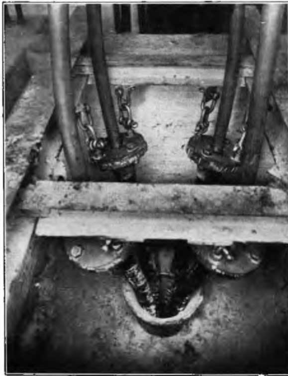
FIG. 5.—CABLE GRIPS OVER BORE TUBE.
