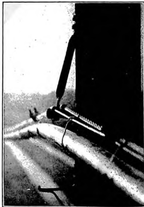
FIG. 5.—CABLE SUPPORTED BY MAIN AND AUXILIARY SUSPENSION WIRES.
