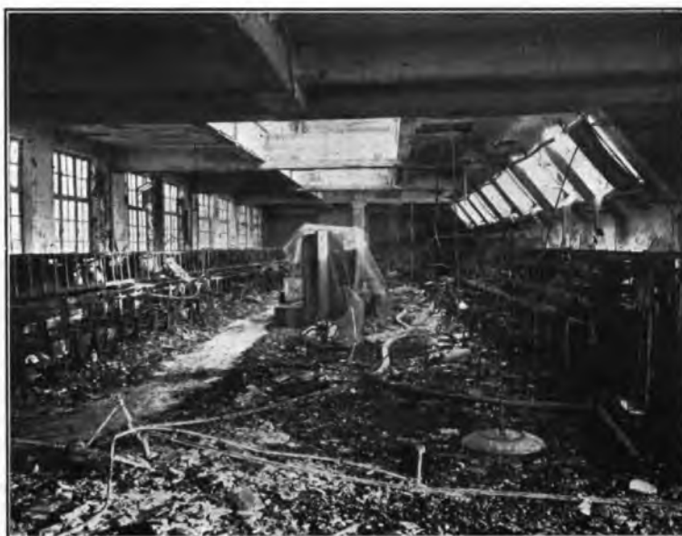
FIG. 3.—AUTO-MANUAL SWITCH ROOM. SIXTH FLOOR.
