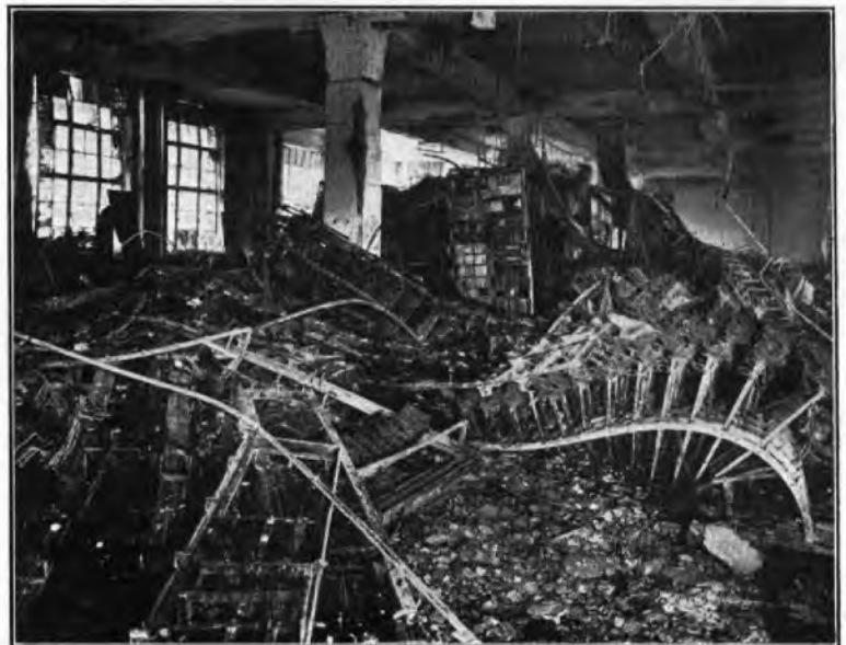
FIG. 1.—I.D.F. GENERAL VIEW OF DAMAGE.
