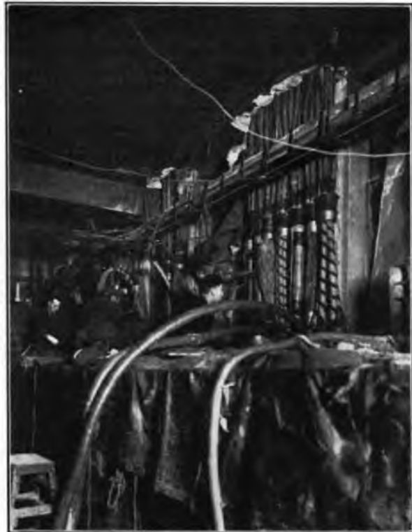
FIG. 4.—PREPARATION OF CABLE TAILS IN BATTERY ROOM BELOW M.D.F.
