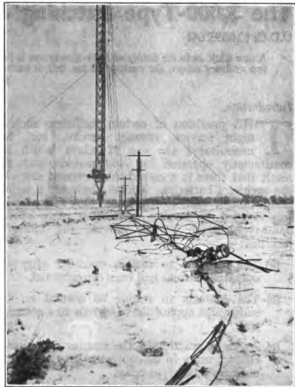
FIG. 4.—GENERAL VIEW OF FALLEN AERIAL.
