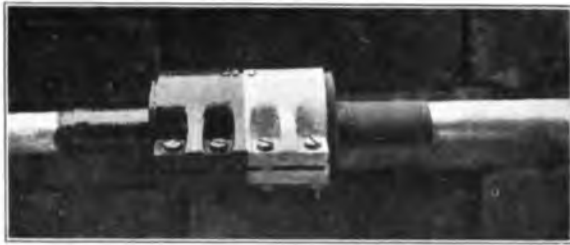
FIG. 4.—GAP COMPLETED WITH METAL COUPLING.
