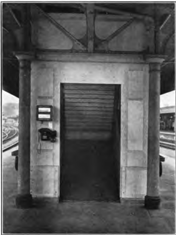
FIG. 4.—DISCHARGE ON RAILWAY PLATFORM FROM TWIN-BAND RISER.
