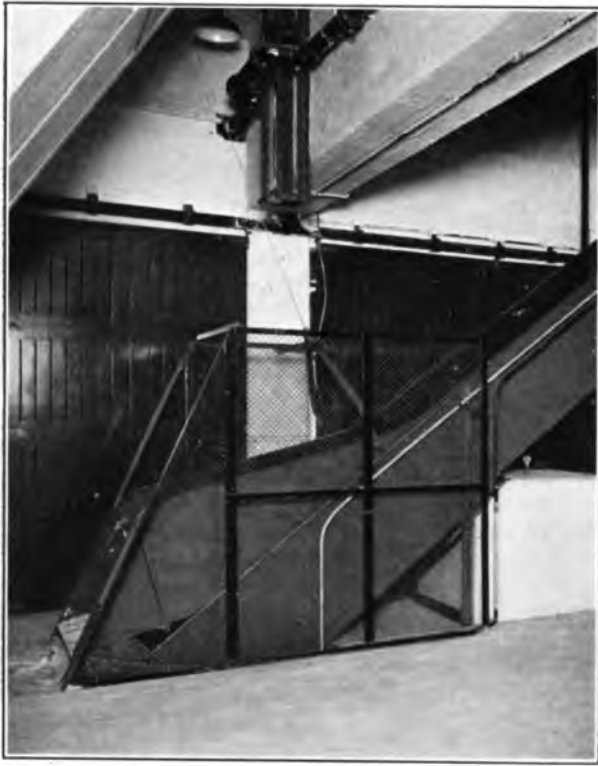
FIG. 12.—HINGED CHUTE FOR OUTWARD LETTER BAG CONVEYOR.
