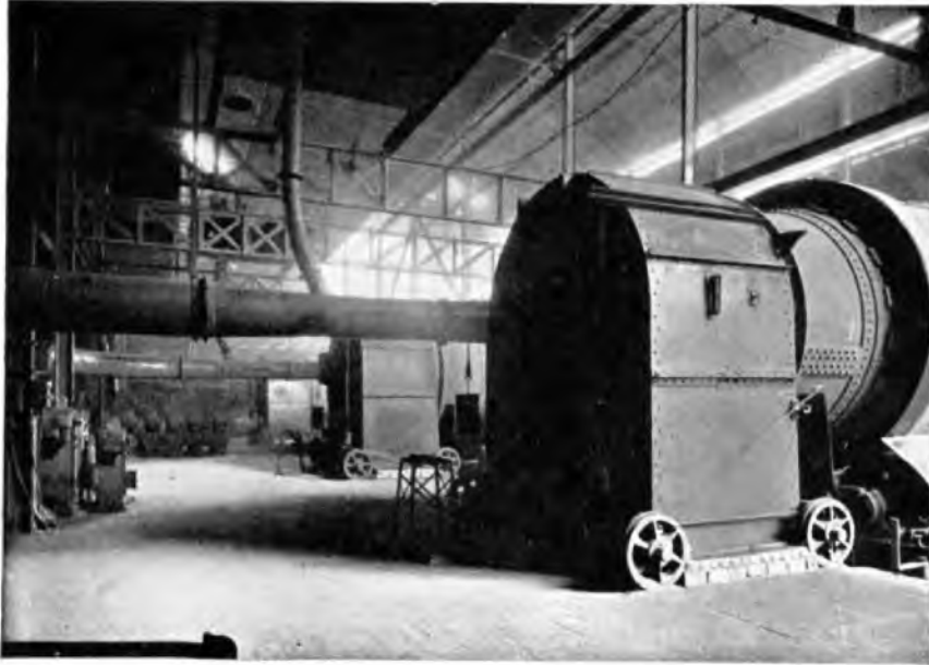
FIG. 4.—FIRING END OF KILNS.
