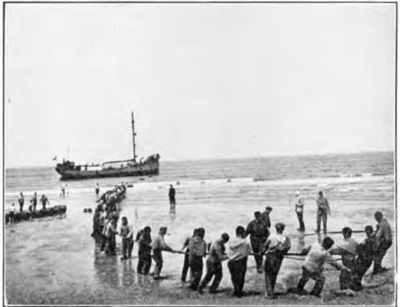
FIG. 2.—LANDING THE SHORE END AT DOMBURG.
