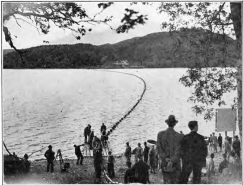
FIG. 5.—FLOATING THE CABLE ACROSS.
