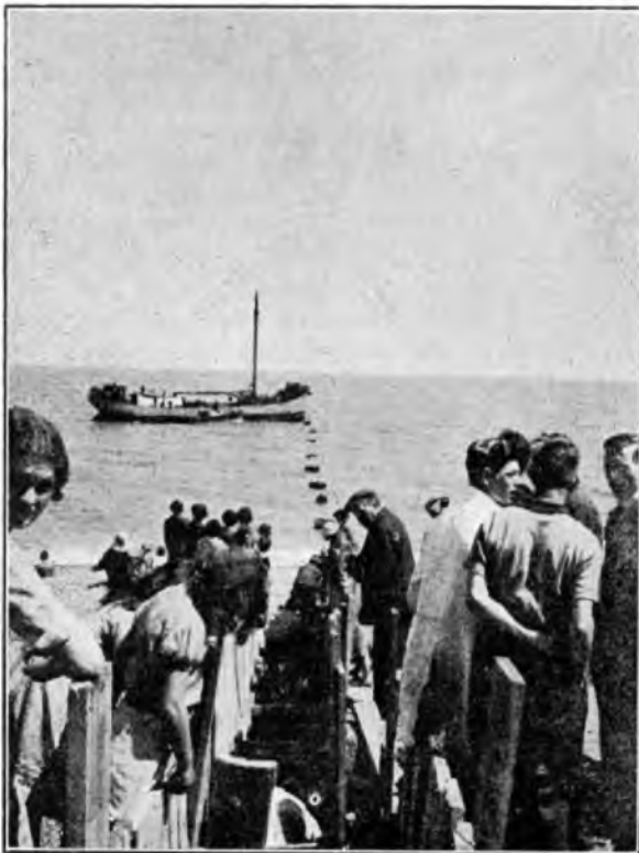
FIG. 1.—LAYING THE SHORE END AT ALDEBURGH.
