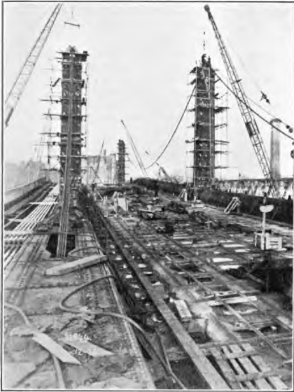
FIG. 1.—VIEW OF BRIDGE UNDER CONSTRUCTION.
