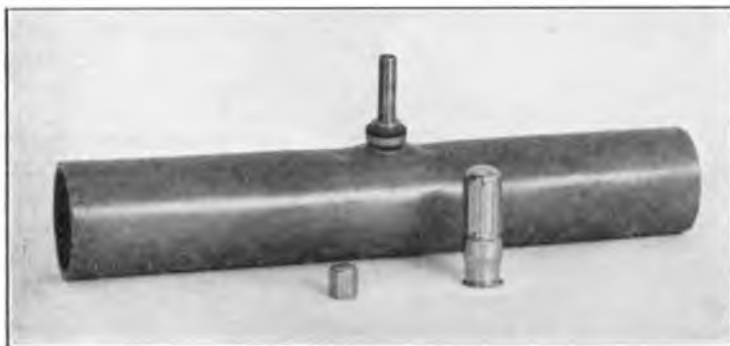
FIG. 2.—SCHRADER VALVE FITTED TO 1½-in. DIAMETER LEAD SLEEVE.
