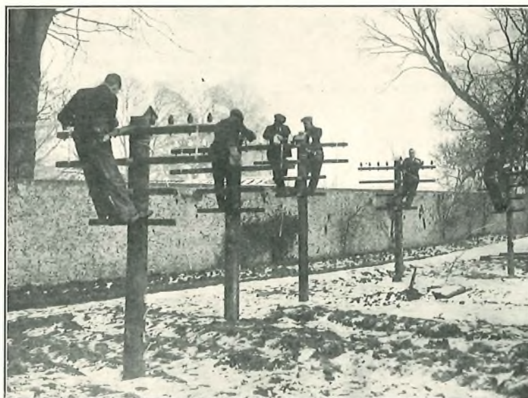
FIG. 5.—EXTERNAL WORK ON SHORT POLES.
