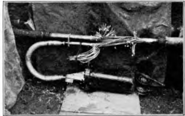
FIG. 4.—LOADING JOINT PARTLY MADE.
