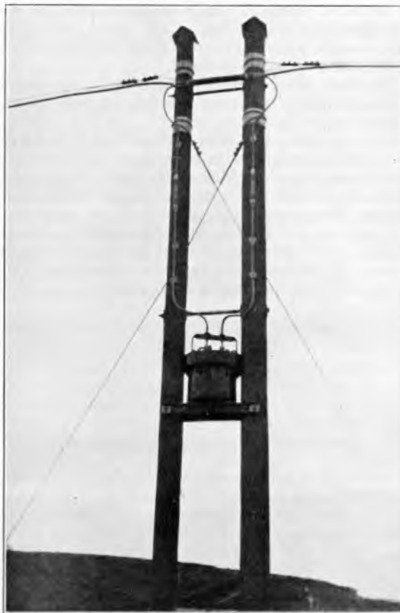
FIG. 1.—AERIAL CABLE LOADING COIL POT.
