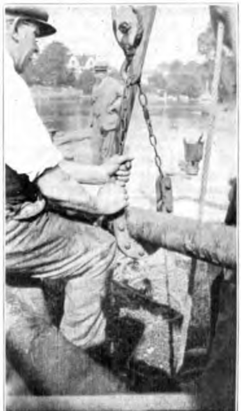
FIG. 5.—PIPE IN STIRRUP SUPPORT.
