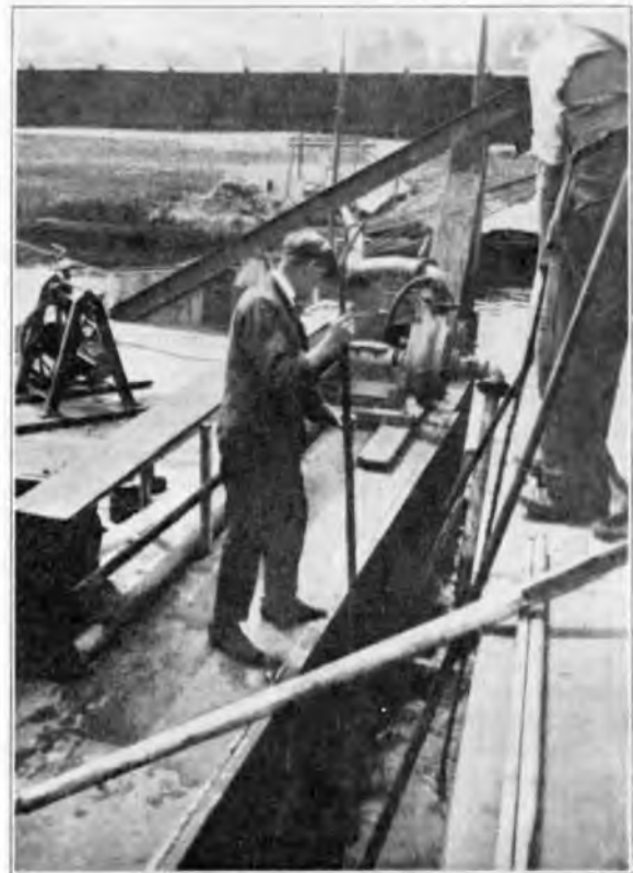
FIG. 1.—MOTOR PUMP MOUNTED ON BARGE.
