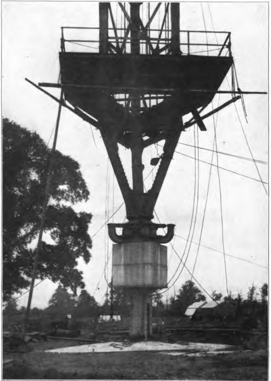
FIG. 1.—BASE OF MAST, SHOWING STEEL STANCHION, GRANITE BLOCKS, PORCELAIN INSULATORS AND BALL SOCKET.
