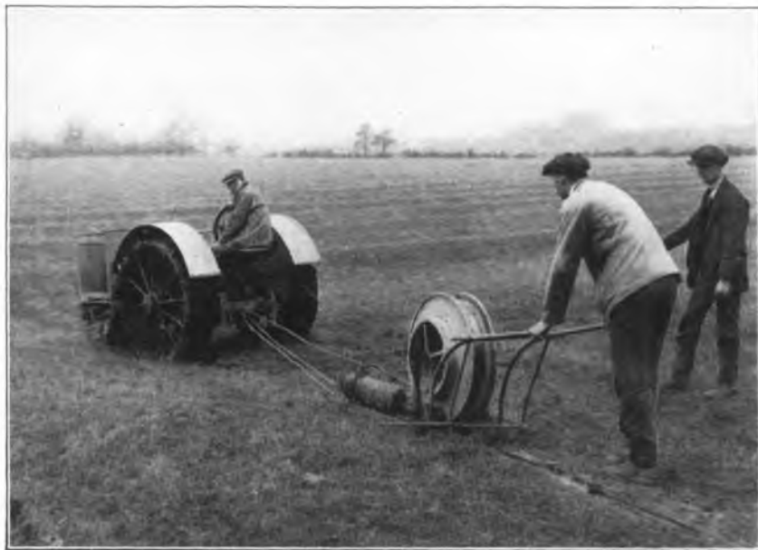
FIG. 4.—WIRE-LAYING PLOUGH.
