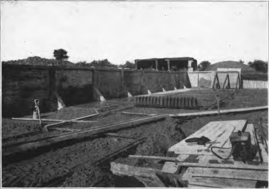
FIG. 2.—500,000 GALLON FERRO-CONCRETE RESERVOIR IN COURSE OF CONSTRUCTION.
