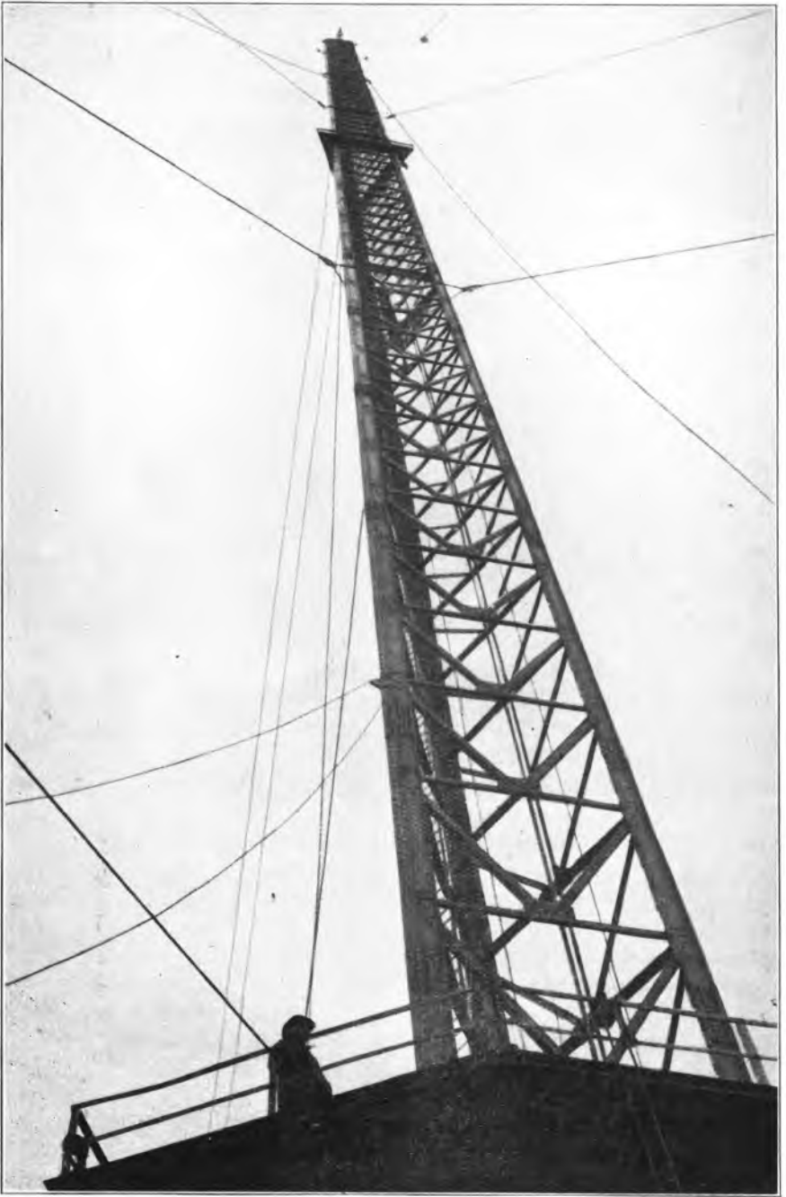
FIG. 5.—ONE OF THE MASTS : LOOKING UPWARD FROM THE GROUND.
