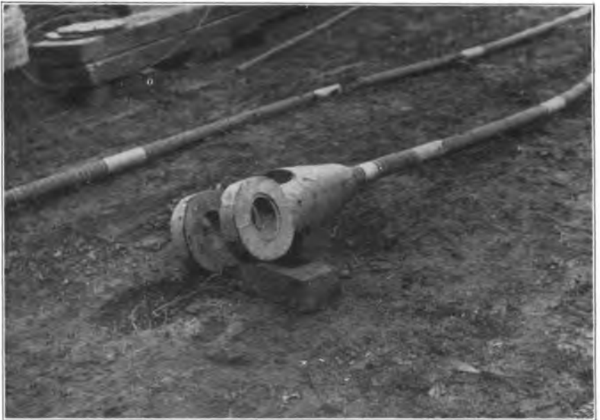
FIG. 3.—SOCKETS AT END OF STAY ROPE.
