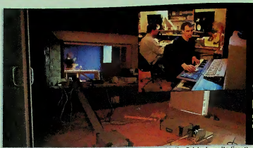
Stanley House's programming rooms under construction, with the finished results (inset)
