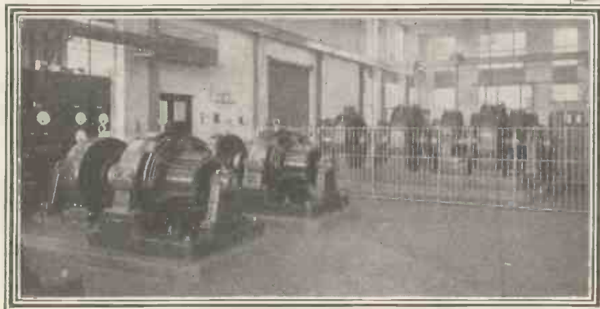
Two of the L.T. generators and the 12,000-volt H.T. generator are shown below.
