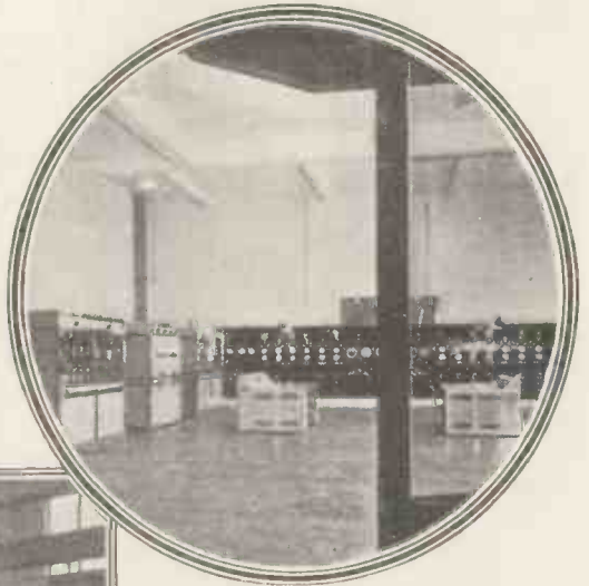
An impression of the main transmitting hall, showing the control desks.
