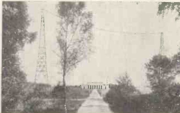
IN SYLVAN SETTING, the transmitter at Motala is found at the end of a long and picturesque drive, typical of the country which it serves so well.
