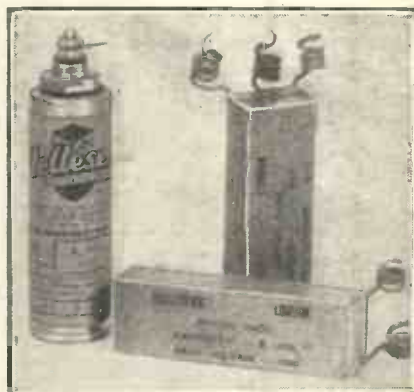
Hellesen wet and dry electrolytic condensers.
