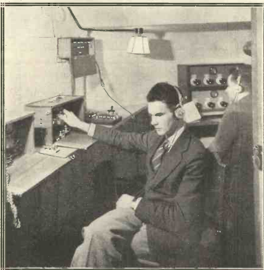
The control apparatus at Queen's Hall is tucked away in a little ante-room between the doors at the main entrance. Throughout the whole of a performance an engineer has to be listening-in or keeping an eye on his programme meter.
