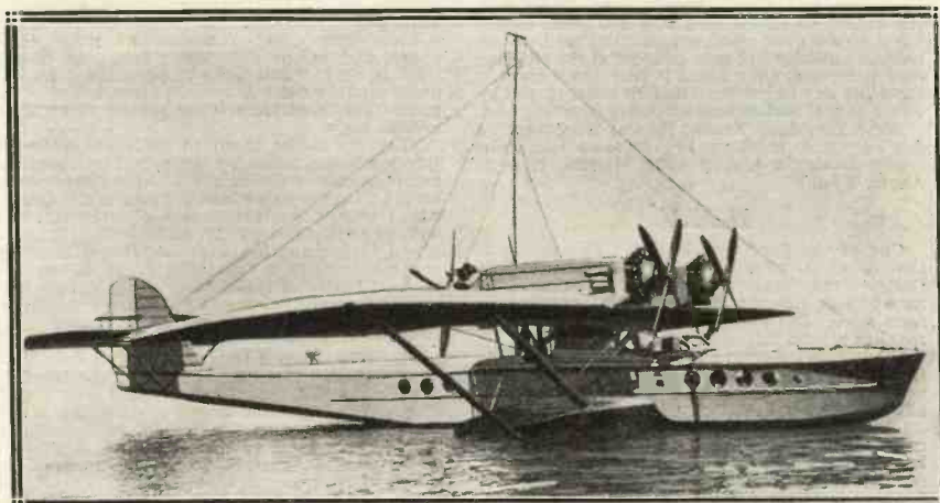
Designed for long-distance cruises, this flying-boat is equipped with a highly efficient radio installation. So that communication can be maintained when on the surface of the water, the aerial is supported on a light mast.
