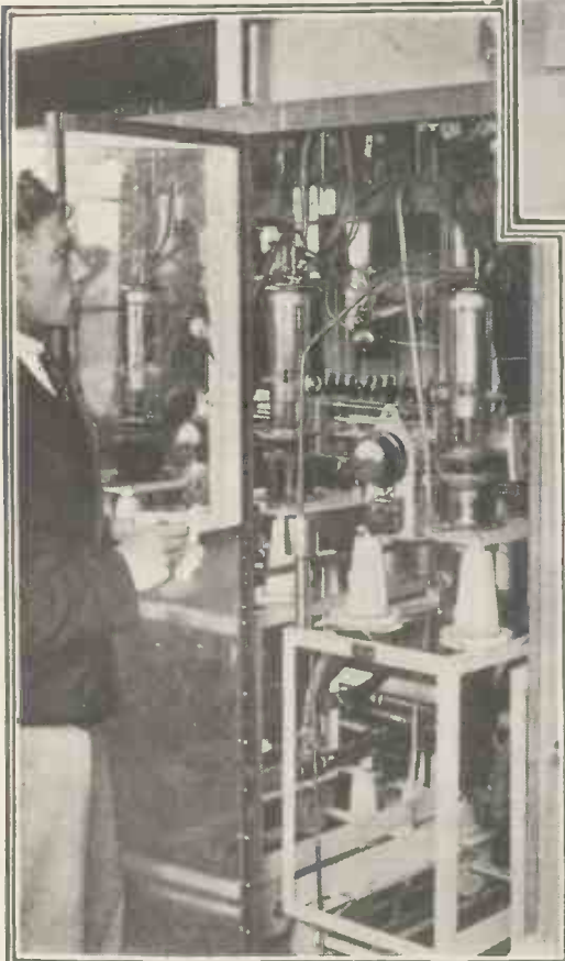
A general view of the aerial system is shown above. The masts are no less than 600 ft. high—the tallest of their kind in the world. The station works on 1,411 metres, developing an aerial power of 160 kw. Below, some of the huge transmitting valves, with water-cooled anodes and filament leads, can be seen.
