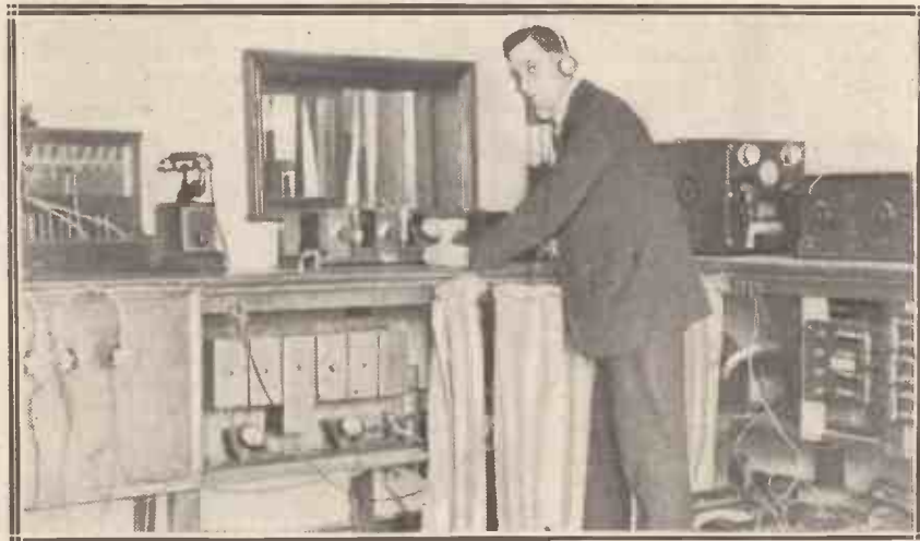
The control room of the Leeds-Bradford relay station, one of the most important sub-stations in Britain.
