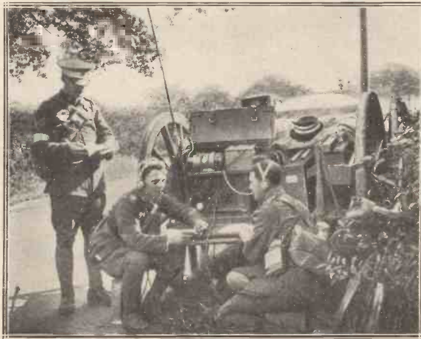
The Signals section keeping an Army Division in touch with G.H.Q.
