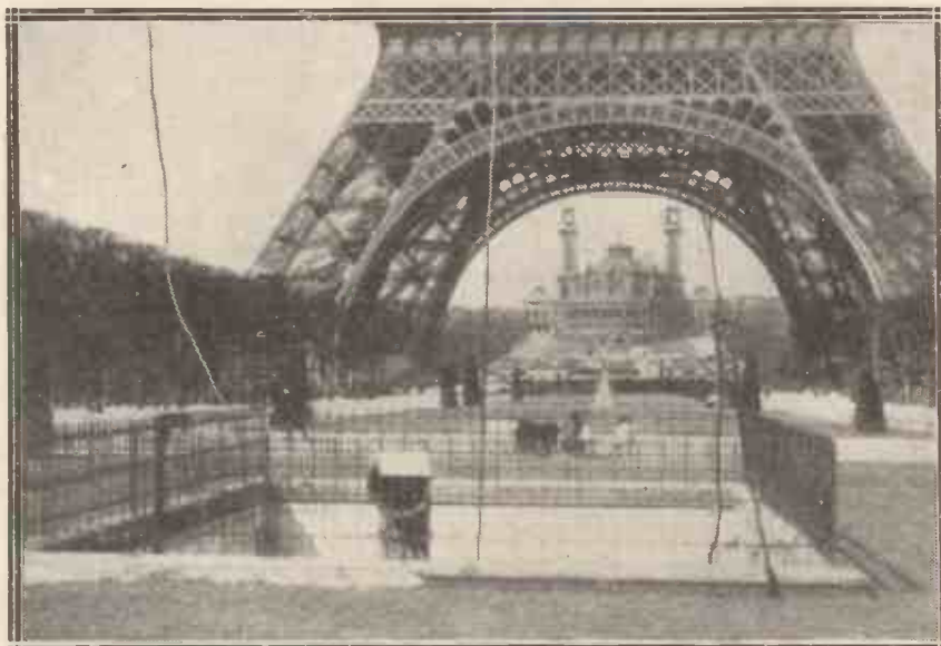
The Eiffel Tower broadcasting station is housed underground, and is famous because it has the highest "mast" in Europe from which to suspend its aerial.
