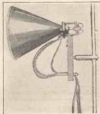
Fig. 2. The "Kathodophon"—a diaphragmless microphone of German origin.
