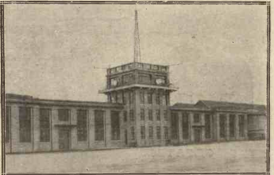
The radio equipment of the Croydon air station is one of the most efficient in the world. Our photograph shows the control tower, where the direction-finding and light signalling gear is housed.
