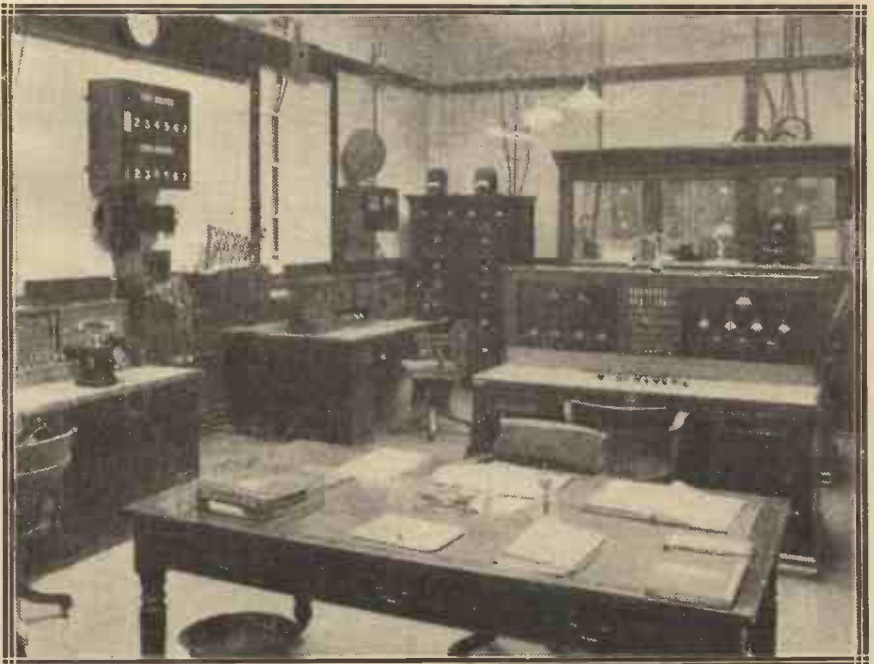
A general view of the control room at 2 L.O.
