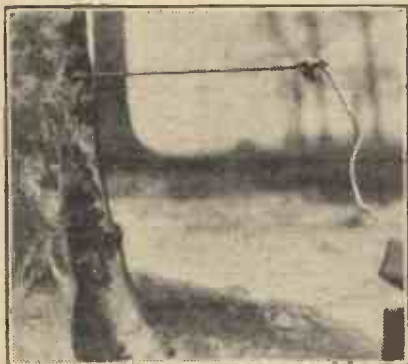
The method of fixing the lead to test a tree aerial.
