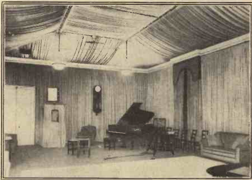
One of the new studios at 2LO, showing the control box.
