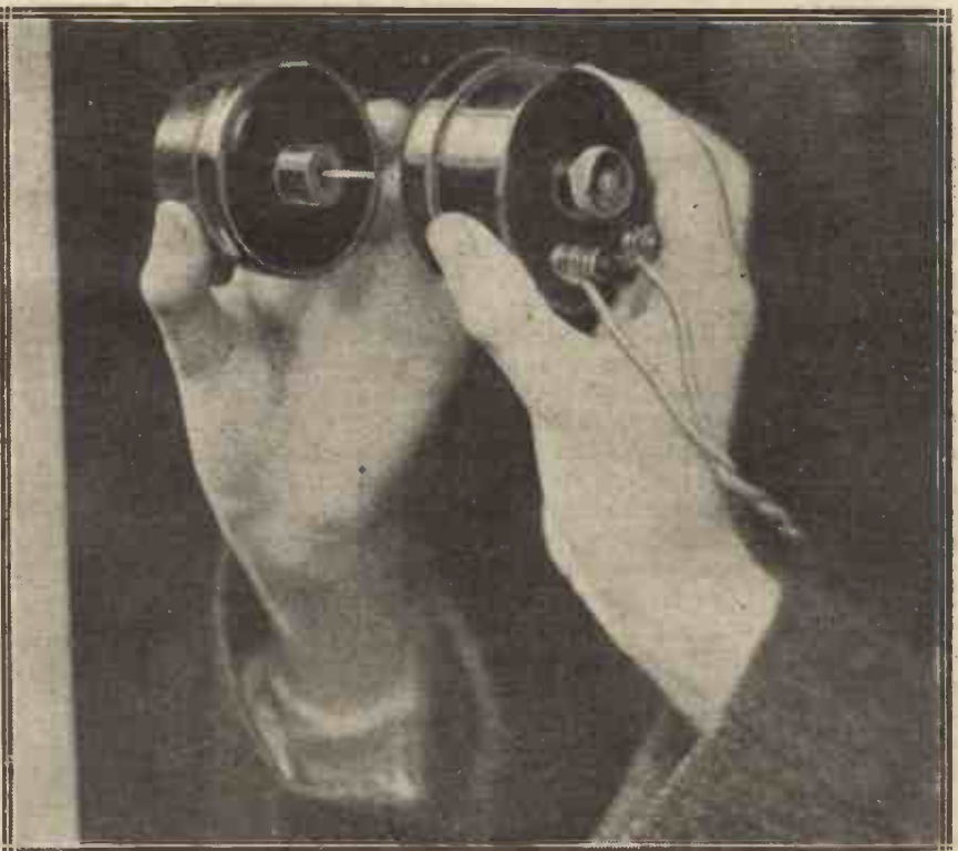
The L.S. Unit was held up to a large mirror when testing the reed movement.
