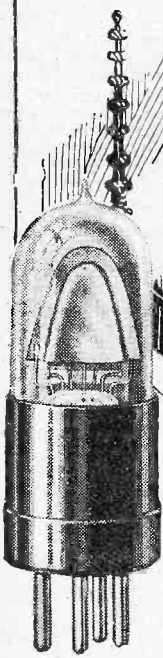
Cossor W.3 Loud Speaker Valve Filament Volts - 1.8 Consumption .5 amps. Price 18/6
