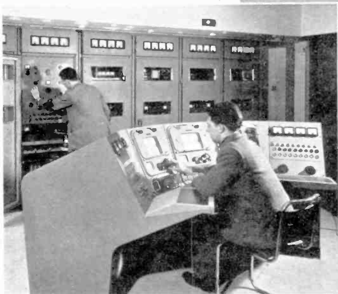
Inside the Kirk o' Shotts TV transmitter, which extended viewing to Scotland. Engineers are adjusting the 5-kW medium-power vision transmitter. The five cubicles at the back contain the vision transmitter. Three similar cubicles (outside the picture on the left) contain the 2-kW sound transmitter. The transmitters are operated by controls on the desk in the foreground. Right: The 750-ft. aerial mast at Wenvoe.
