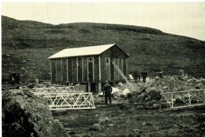
Fig. 9. The Torneträsk Translator Station during erection.
