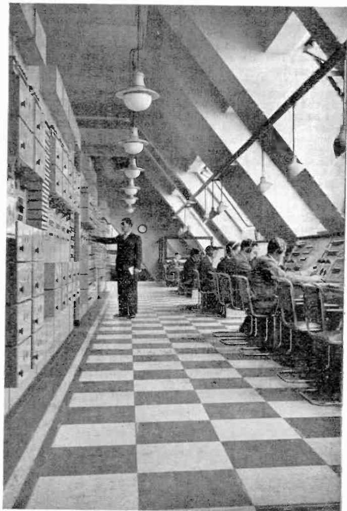
CONTROL ROOM, BROADCASTING HOUSE
