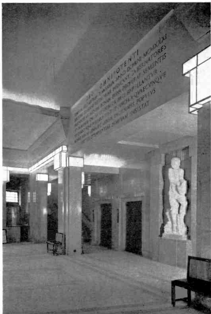
ENTRANCE HALL, BROADCASTING HOUSE
