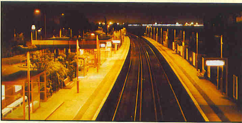
Photo 6. Southampton Parkway Station. Full cut-off lamps installed to prevent glare to train drivers. Camera position shows effectiveness of luminaires; not visible in picture. ©Copyright R. Arbour.
