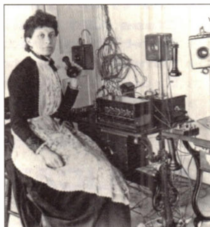
An operator at the early Croydon exchange. Photo reproduced by kind permission of BT Archives. © 1992 British Telecommunications Plc.
