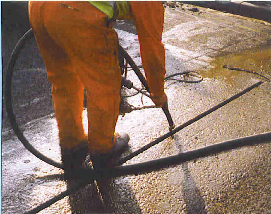
Top left: An installation engineer cutting out a slot for a strip sensor.
