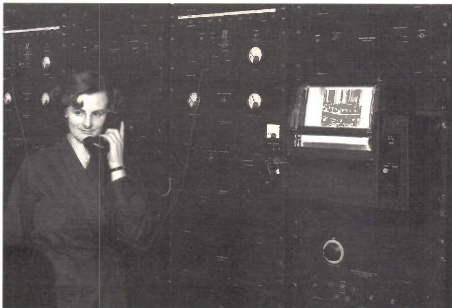
The 1951 Muirhead ‘Mufax’ equipment in use, showing the control panel.
