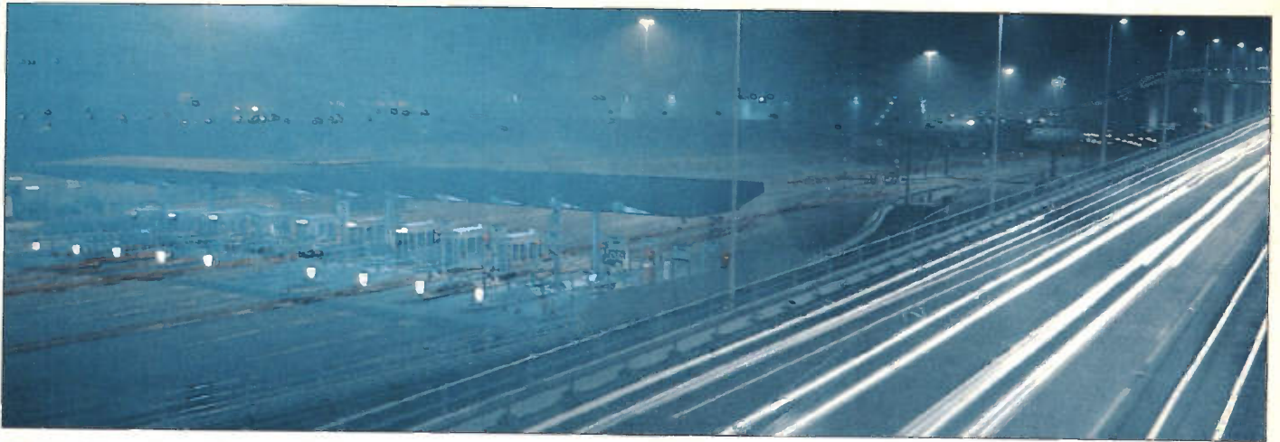
QEII Bridge and northbound toll plaza at night.
