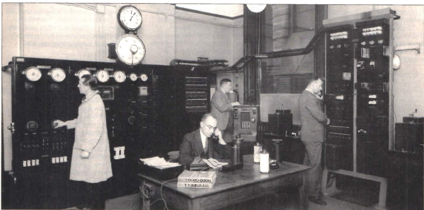
In 1930, the Post Office opened a 'Picture Telegraphy' service initially to Berlin. Using Siemens-Karolus equipment, the sending and receiving machines are either side of the control panel on the right.
