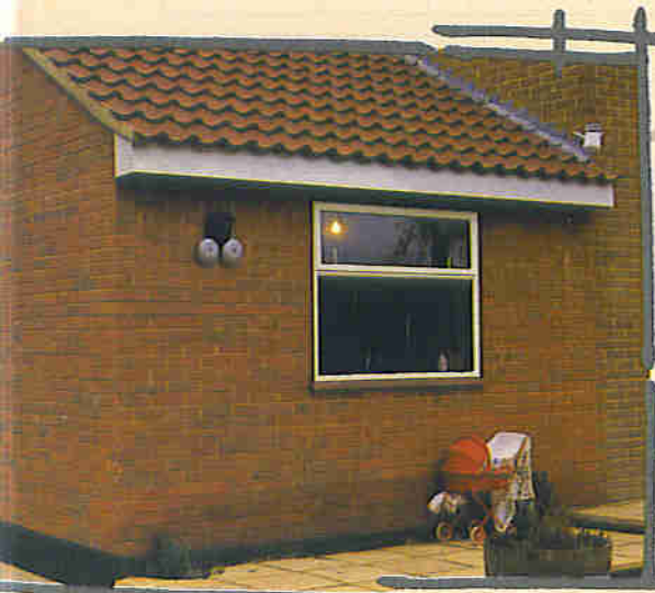
House extension in which Ian installed an external telephone bell, and PIR operated security light.
