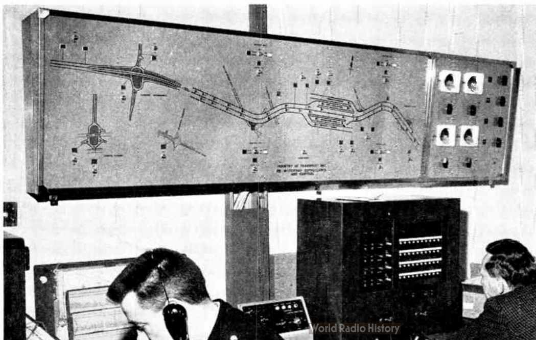
This shows the mimic diagram installed at Hounslow Police Station
