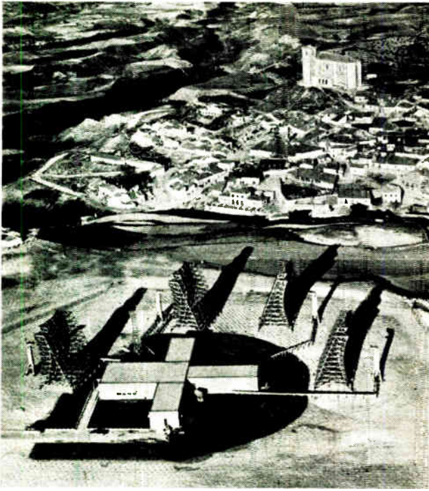
Located near Humosa in Northern Spain, this troposcatter aerial array serves one of the stations providing multi-channel voice and teletype service for U.S.A.F. operations in Western Europe extending from England across the Bay of Biscay through Spain. The span from England to Spain utilizes the highest power amplifiers ever to be incorporated into a troposcatter system. The aerial and feed horn structures for Humosa and other sites were fabricated and hot dip galvanized by Painter Brothers Ltd., a member of the B.I.C.C. Group
