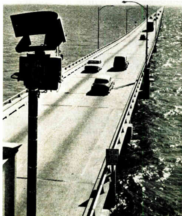
This radar aerial (left) looks out over world's longest causeway spanning the 24-mile-wide Lake Pontchartrain near New Orleans, Louisiana. Raytheon radars and marine radiotelephones have been installed at the two bascule bridges, eight miles out from each shore, where ships cross the roadway. To safeguard motorists who 'go to sea' in their cars in foggy weather, causeway personnel keep a radar watch for loose barges or disabled vessels that might stray from regular ship channels and drift towards the bridge
