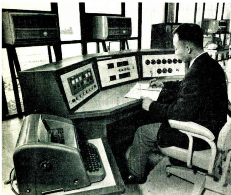
The control console which is situated in the computer room
