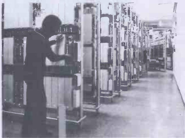
A typical Strowger exchange using contacts which rotate past banks of contacts.
