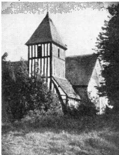
Fig. 2—Same negative, but the tower 'rescued' by enlargement
