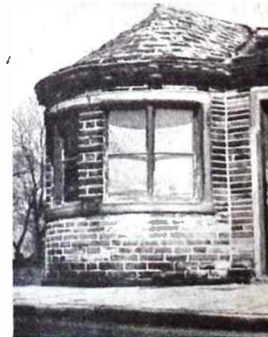
This old toll house at Bradford was demolished five years ago, but was photographed for record purposes before it disappeared.
