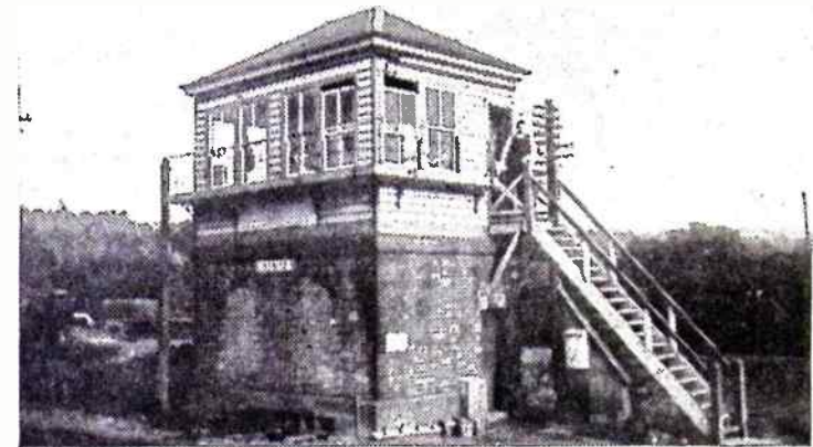
Typical S.E. and C.R. signal box, Merstham (S.R.)
