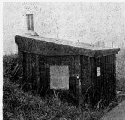
A typical Platelayer's Hut
