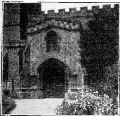
A DISMAL FAILURE.
