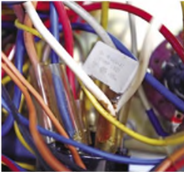
This mains capacitor in the voltage selector fails and produces smoke. The one here is a replacement.
