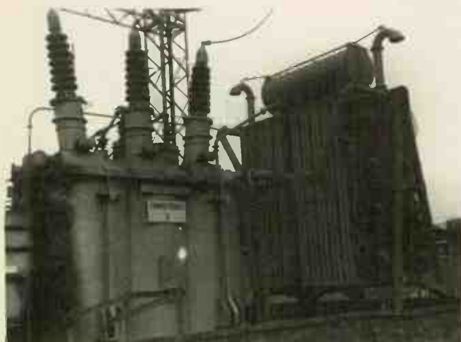
Putting hi-fi in perspective - if a 500VA transformer sounds chunky, then try 90000000VA as used by electricity companies!
