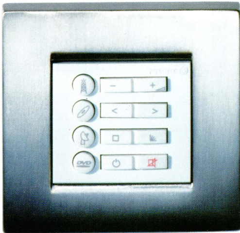
Individual control panels are sited in each room and come in a variety of styles and finishes to suit (nearly) any interior.
