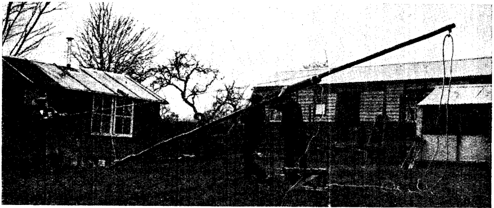
Fig. 3. Two of the men helping to erect the double mast in the photograph are making use of the guy-ropes. By this means the mast is prevented from swaying
