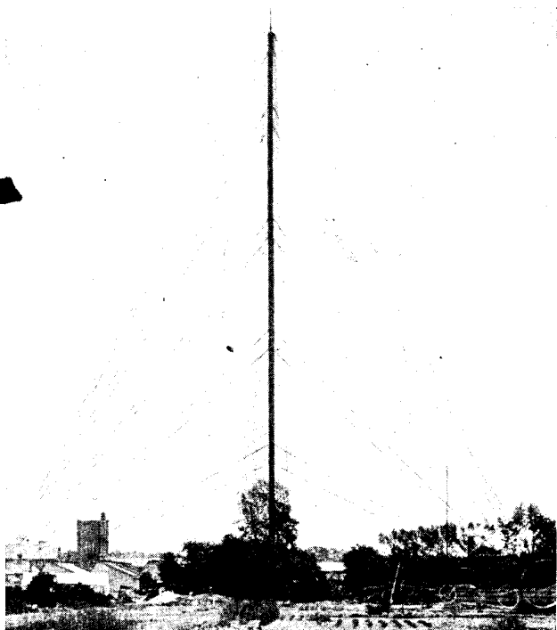
STEEL MAST AT CHELMSFORD
