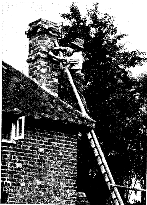
Fig. 2. In order to prevent the ladder from slipping sideways the top is placed across the corner of the chimney stack in this case
