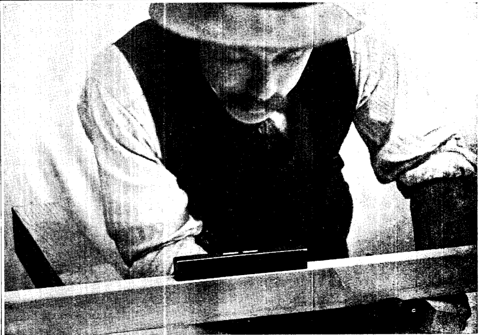
Fig. 1. One of the most useful instruments for the wireless experimenter who carries out his own woodwork construction and makes his own cabinets is the carpenter's level here seen in use. This pattern of level is usually 9 in. long and is inexpensive
