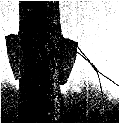
Fig. 3. An efficient way to guy a mast is by fastening wooden chocks on it and forming a loop or a bight in the guy, as shown
