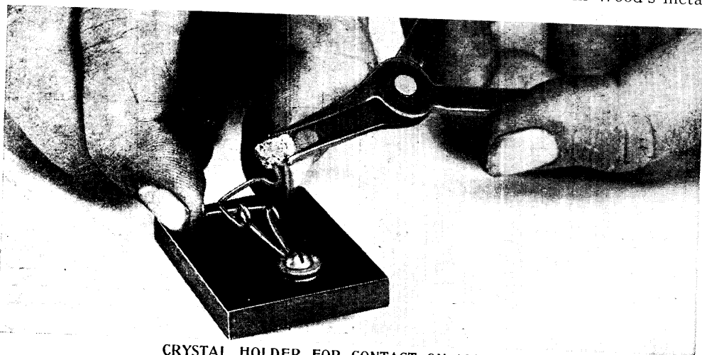
CRYSTAL HOLDER FOR CONTACT ON ALL SIDES
