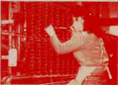
TELEPHONE EQUIPMENT. Ersin Multicore being used to solder switchboard apparatus at Autelca Mediterranea, S.A.T.A.P.—one of Italy's largest manufacturers of telephone equipment.
