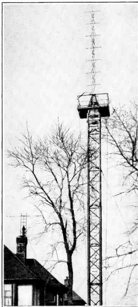
The "turnstile" aerial at W2XCR, formerly W2AG, the 600-watt, 110-Mc/s station of C. R. Runyon, at Yonkers, New York, which uses Major Edwin H. Armstrong's system of frequency modulation. Articles in the May 11th and 18th issues of "The Wireless World" describe reception tests on some of the twelve American stations using frequency modulation.
