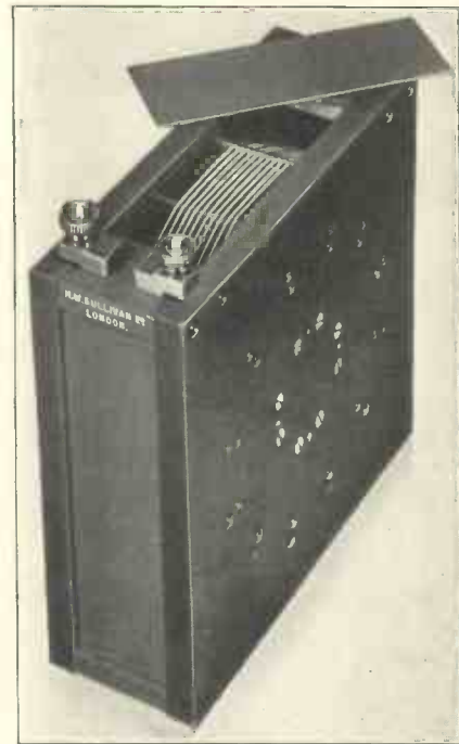
Fig. 2.—Sullivan-Griffiths thermal compensated inductance; multi-layer type.
