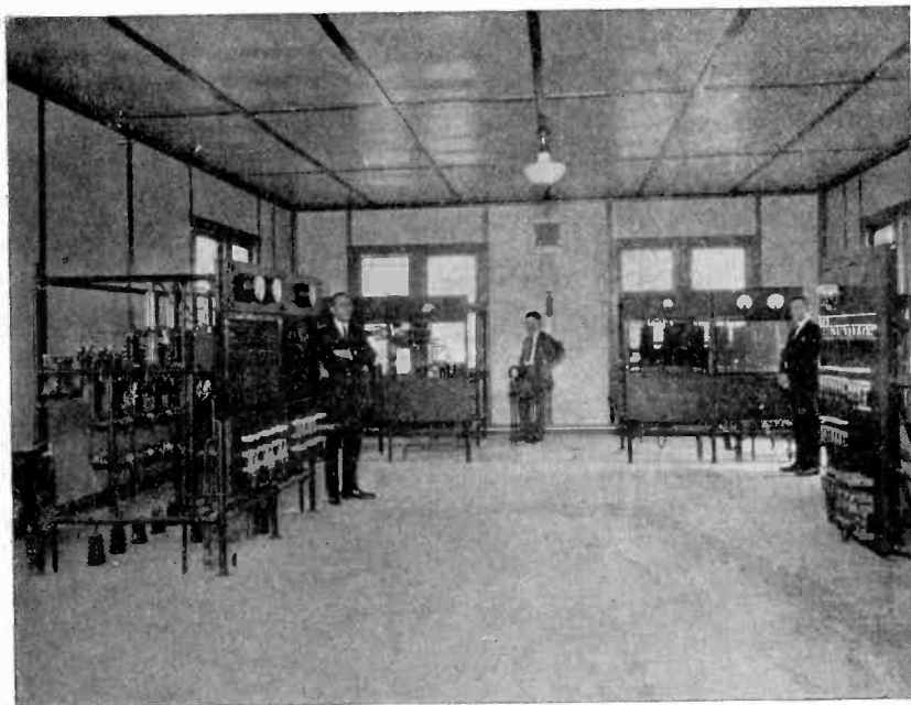
The Interior of the Control Room at KDKA (see p. 304.)
